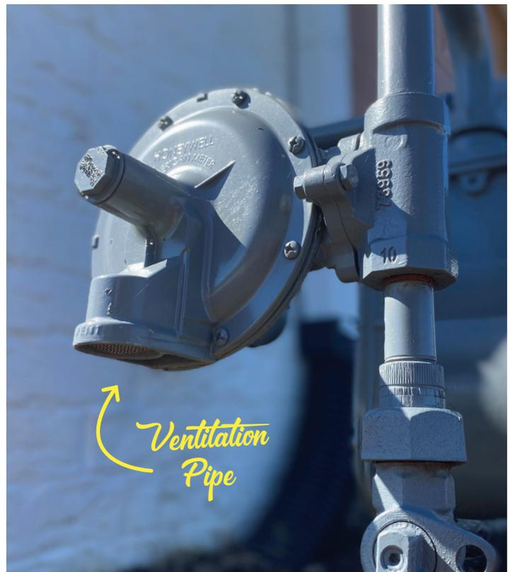
Be sure to *gently remove* all snow and ice buildup from the meter and ventilation pipes. The ventilation pipe is located underneath the saucer shaped portion of the meter equipment.
